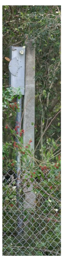
Photo #2 This is a composite photo showing the smaller pole that is adjacent to the power pole in front of the eagle nest. It is about 8-10 feet tall. Note the wooden switch handle protruding to the left, and the electrical conduit emerging from underground. This structure is located on City of Pembroke Pines property. It looks quite old, perhaps a remnant from the former owner of the property. The fact that the power pole contains a transformer suggests that a service line is (or was) in place.
